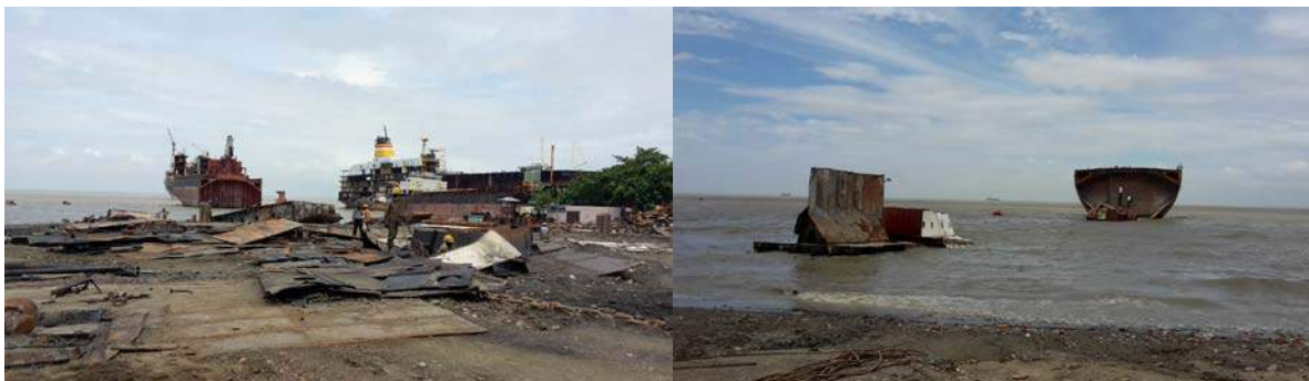
Figure 4: Chittagong ship recycling yards (Source : Sofies SA)
